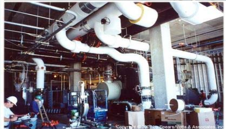
Trigen/Inner Harbor East Heating and Cooling Plant in Baltimore. (Photo credit: Spears/Votta & Associates.)
