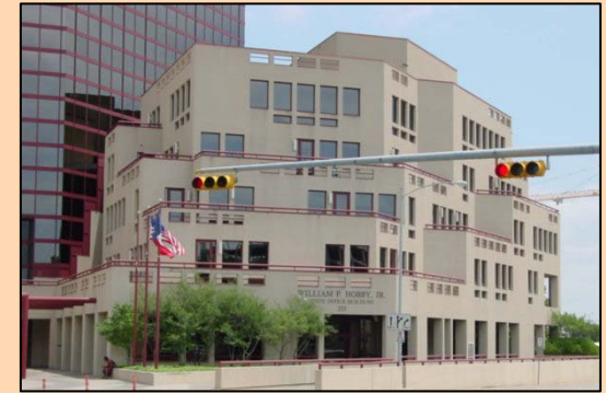
Hobby Office Bldg.
