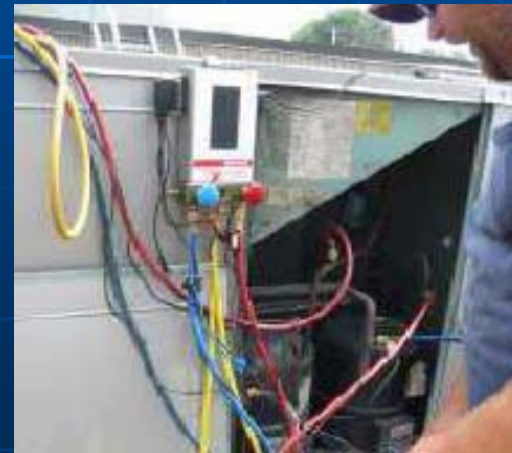
4. Re-test and document post repair state
