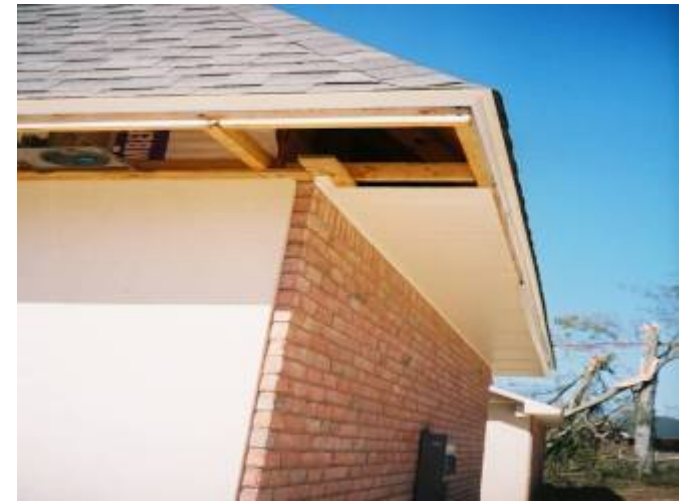
Soffit failure = water entry
