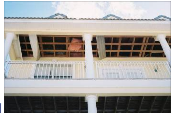
Soffit failure = water entry
