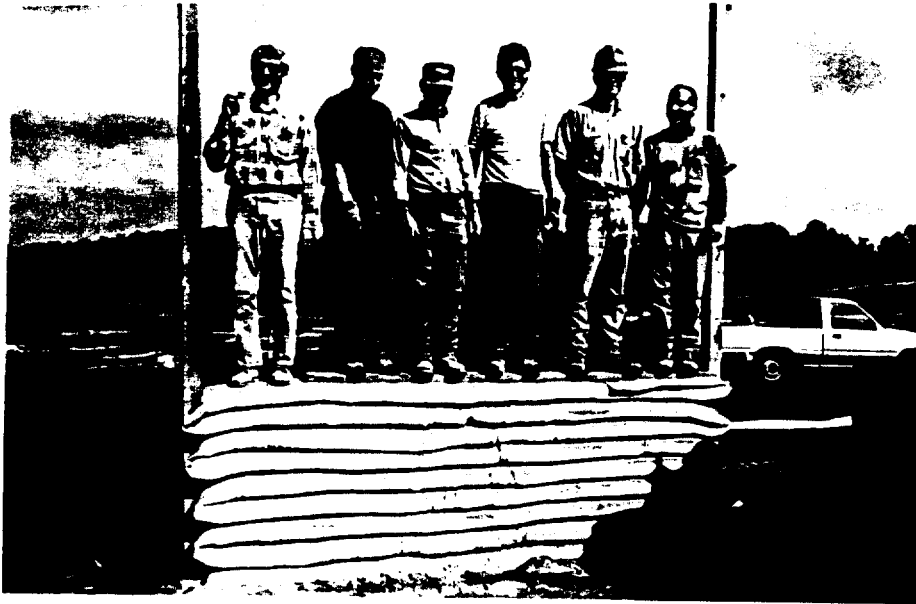
Figure 5. QuickFill fly ash wall before it is covered with wire mesh and stucco.
