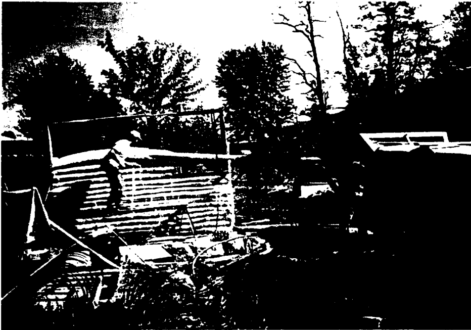
Figure 6. QuickFill sawdust wall. Sawdust is sucked out of the trailer and blown into the fabric tube.
