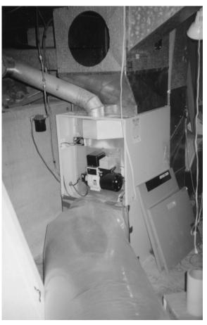
foam plugs from the registers and air handler unit, cover and seal any holes cut in the ducts with sheet metal and mastic, reinstall fans and covers, and reinstall any air handler units that were removed.
