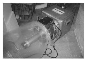
Figure 2. The Aeroseal Tubing Connection
