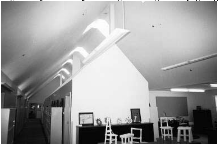
Figure 1. Quabbin Project – Integrated Ridgeline Skylighting
