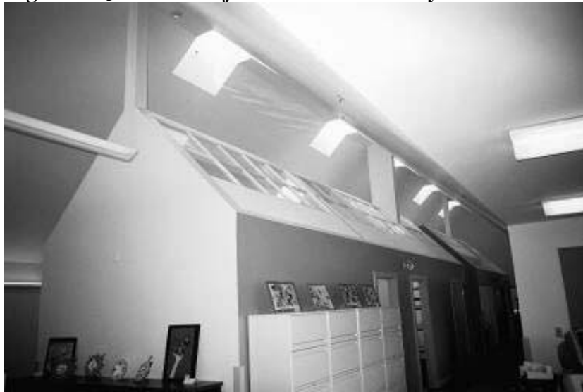
Figure 2. Quabbin Project – Interior Roof System
