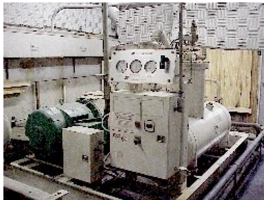
Figure 4. Allegheny Rodney Primary 125HP Rotary Screw Compressor
