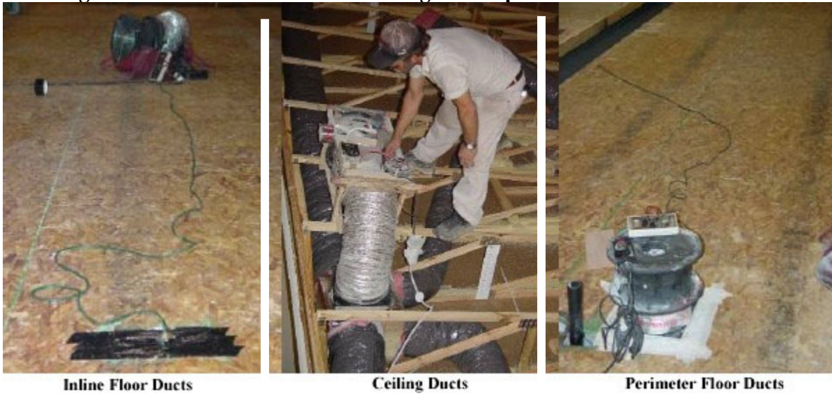
Figure 4. In-Plant Duct Blaster Testing – Incorporated into Production Line
