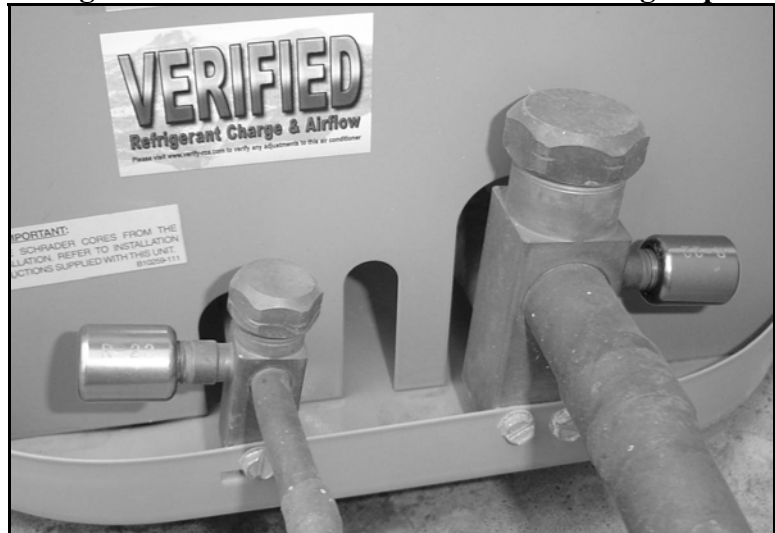
Figure 9. Verified RCA Sticker and Locking Caps
