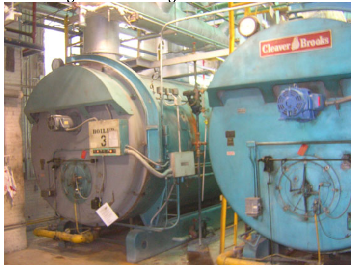
Figure 1. Existing Steam Boiler Plant
