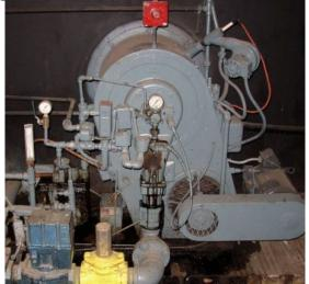
Figure 3. Burner's Linking Mechanism
