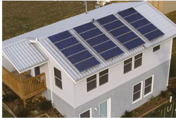
Figure 2. ZEH4, 1200 ft 2 with 2 Ton 17 SEER Air-Source Heat Pump
