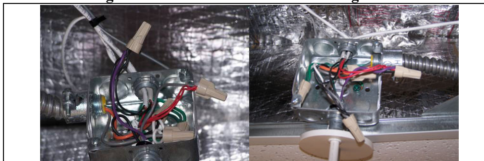
Figure 8. Incorrect Photosensor Wiring
