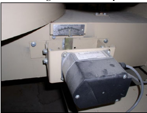
Figure 8. Combustion Air Damper in Linkageless Control System
