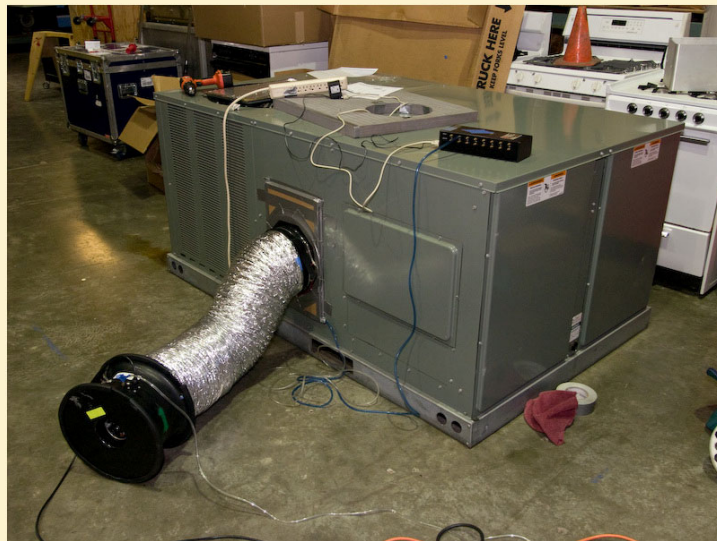
Figure 1. Roof Top Unit Undergoing a Pressurization Test
