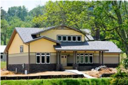
PCM House at 100 Cross Creek Place
