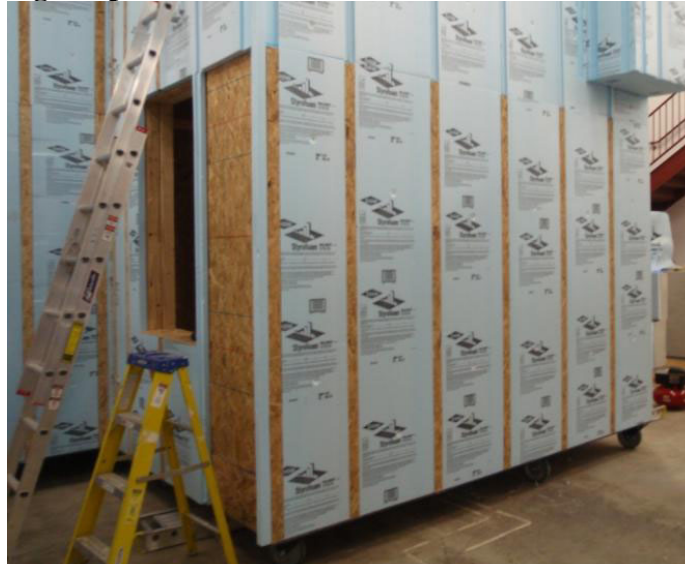
Figure 3. Furring Strips Installed in Recessed Channels of Insulating Sheathing
