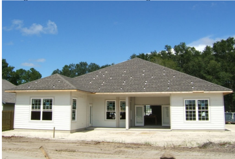
Figure 2. Home at Dried in Stage of Construction
