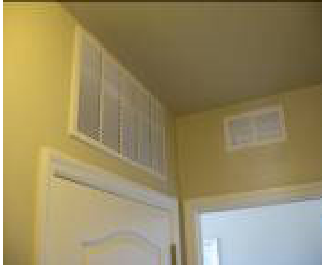
Figure 7. Air Handler in Conditioned Space
