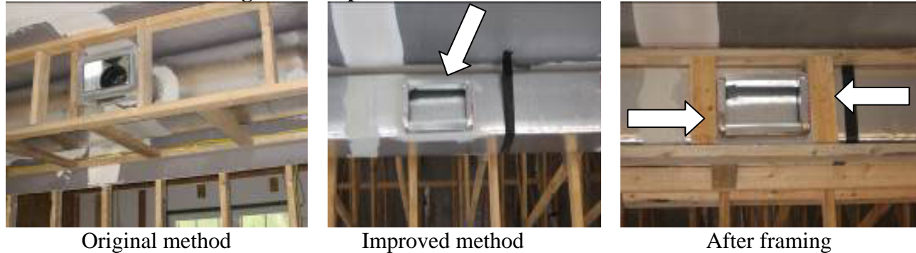
Figure 5. Improved Method for Duct Installation
