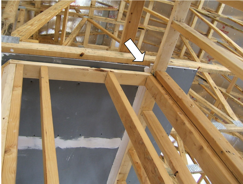
Figure 3. Drywall Installed Between Top Plate and Bottom of Roof Truss
