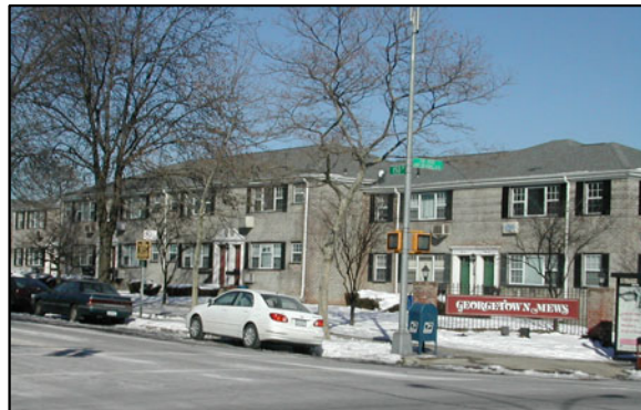
Figure 1. Georgetown Mews Complex
