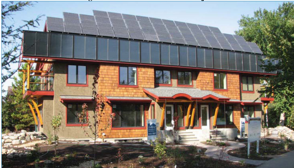
Figure 3. The Riverdale NetZero Project
