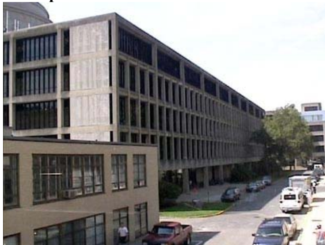
Figure 2. Views of the MIT Materials Science Building, Building 13, which MIT plans to have ISO 50001 Certified
