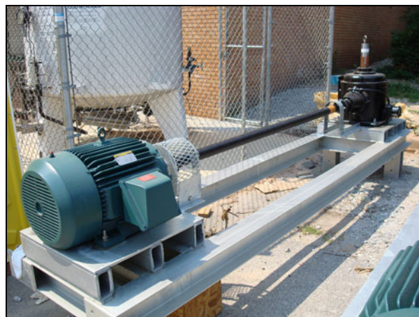
Figure 2. Typical Fan Drive Arrangement
