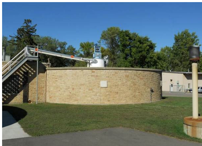
Figure 1. Anaerobic digester with a new mixing system
