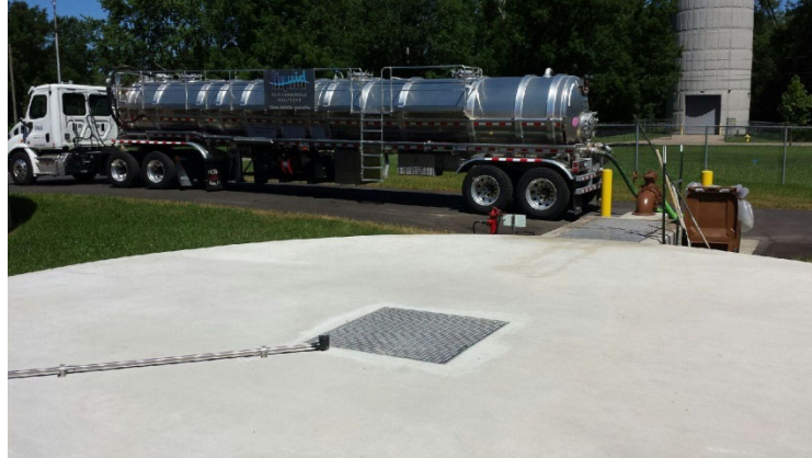
Figure 4. Receiving station accepting trucked in material
