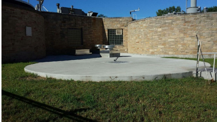
Figure 3. Waste receiving station
