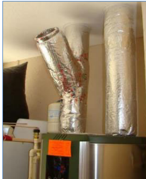
Figure 8. Ducting arrangement at Site 5 allowing cold exhaust air to be diverted from the conditioned living environment if comfort became an issue during winter.
