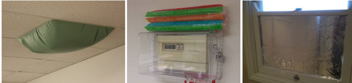
Figure 2: 2A: a bag placed over vent to prevent air movement; 2B: popsicles placed on thermostat to “trick” settings, and 2C: aluminum foil placed over window. Source: author’s photograph & google images.
