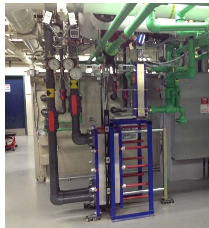
Seawater Heat Exchanger
