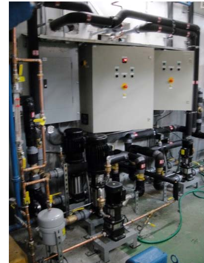
Hot Water Piping
