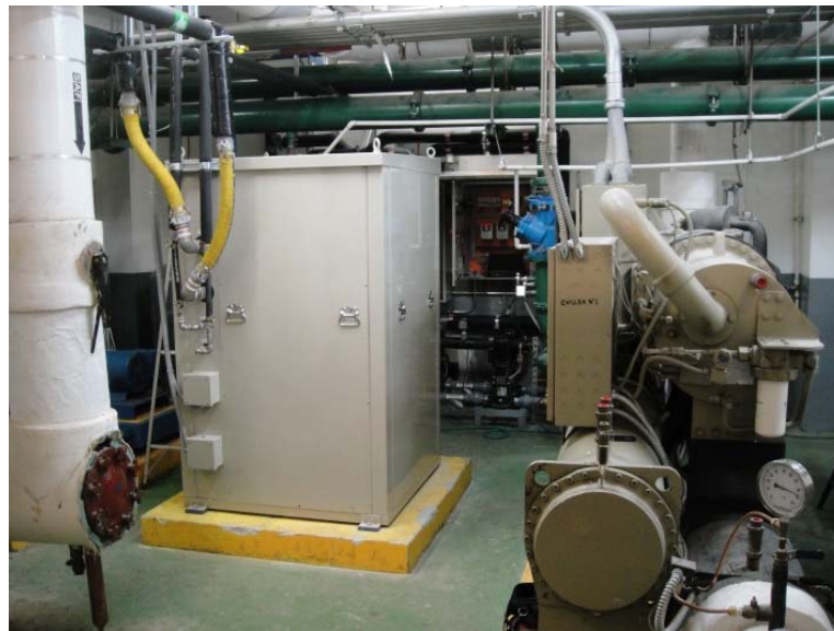
Heat Pump installed in chiller mechanical room
