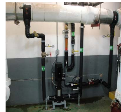
Heat Source Piping
