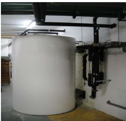
Hot Water Storage Tank
