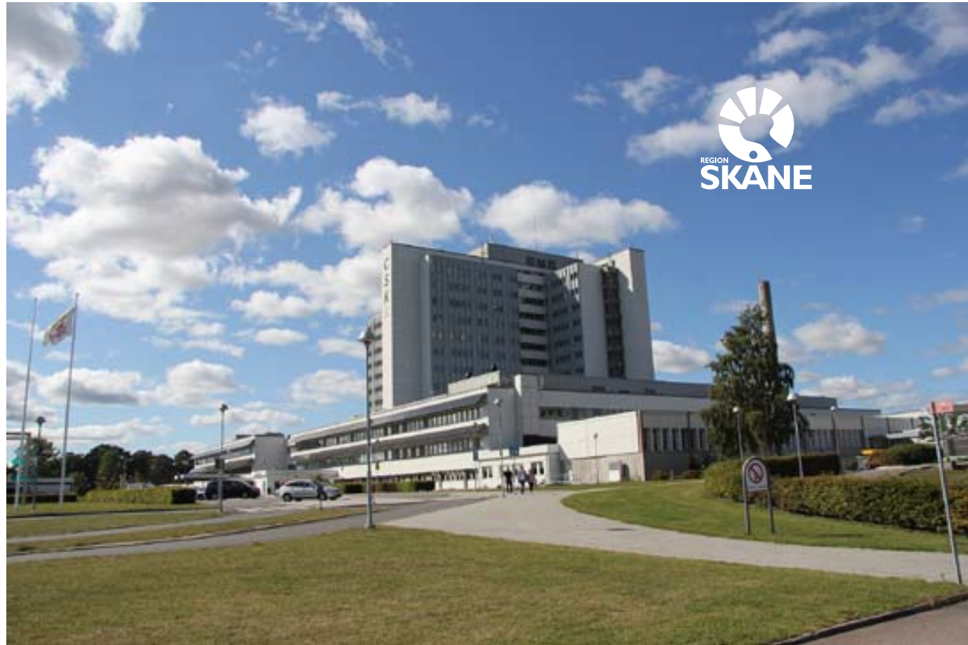
CENTRALSJUKHUSET KRISTIANSTAD FIRST INSTALLATION IN THE HEALTHCARE SECTOR
