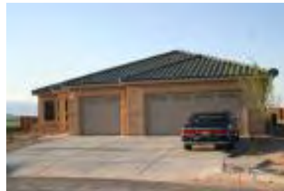
LEED-certified home in Los Lunas, NM Photo credit: Artistic Homes
