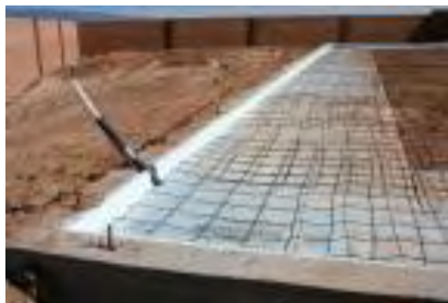
R-10 full perimeter slab insulation Photo credit: Artistic Homes
