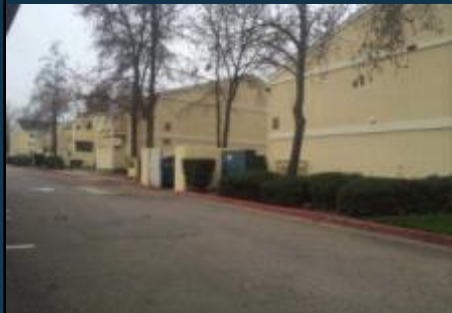
Madison Blvd– 86 units
