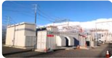
Distribution Level Energy Storage
