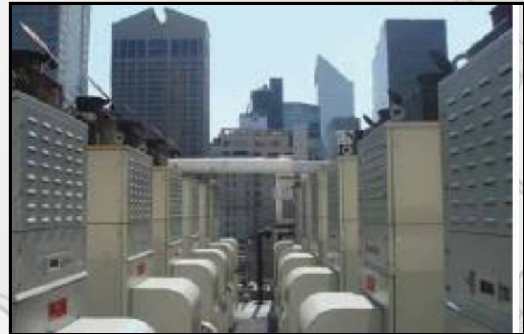
Commercial CHP installation
