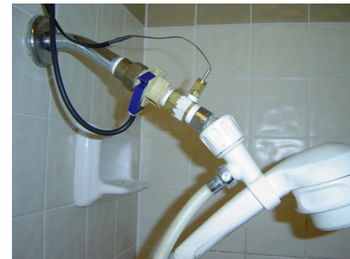
LBNL system captures time, temp and flow at shower and transmits data wirelessly to server database
