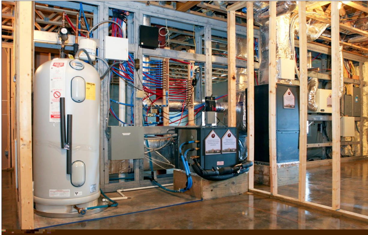
Separate Units [Water Heating; Heating/Cooling]
