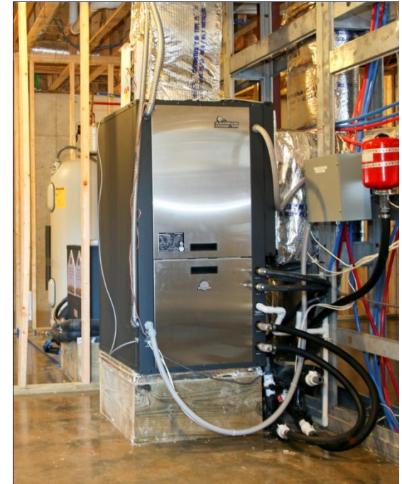
Single Unit [Water Heating; Heating/Cooling]
