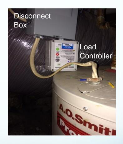
Mosaic adds a load controller on the electric line to each water heater
