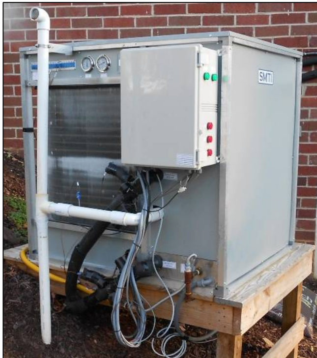
Beta 1 GAHP installed at home in Northeast TN
