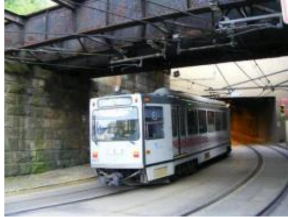
Vehicles as sensors for infrastructure assessment
