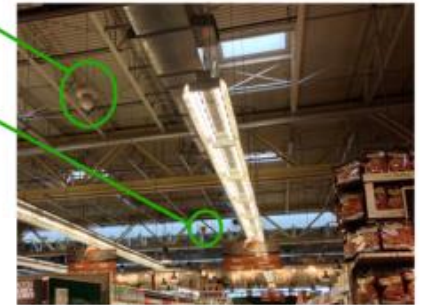
Speakers as sensors for indoor localization
