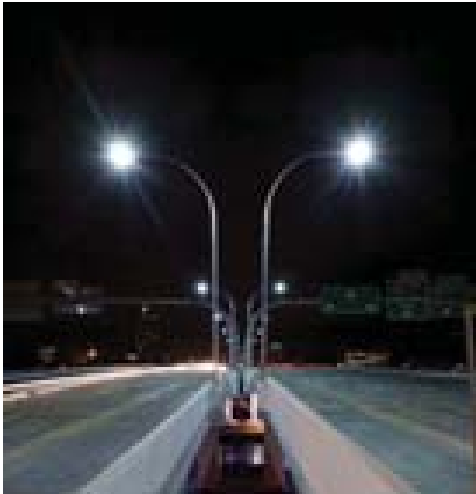
LED Lighting on I-35W Bridge, Minneapolis. Source: DOE.
