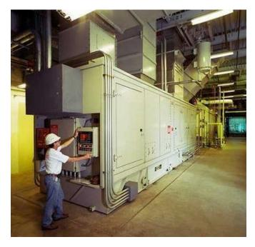
Figure 4. Gas turbine CHP system at Bristol-Myers Squibb in Wallingford, CT. Image courtesy of DOE/NREL. Credit: Bernard Blessinger.
