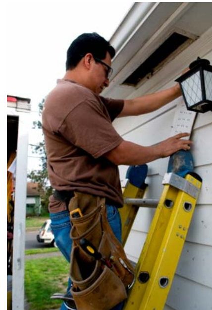
A CEWP contractor installs attic ventilation in accordance with Building Performance Institute standards. Courtesy of CEWP.
