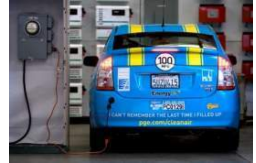
Smart charging for electric vehicles
