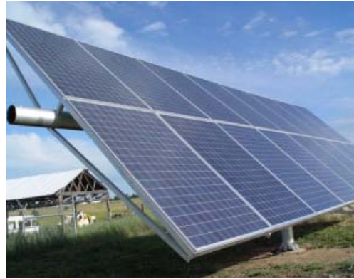
On-site generation and storage
