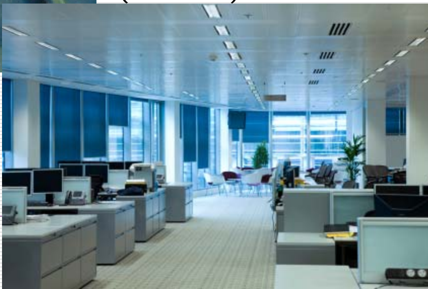
Commercial Lighting (Coml EE)
