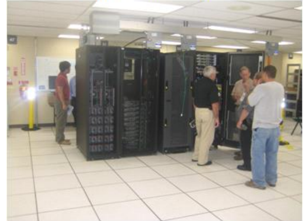
Duke Energy 380VDC Data Center Demo
