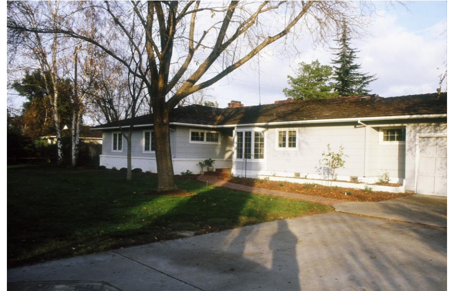
Retrofitted Home: High-Performance
