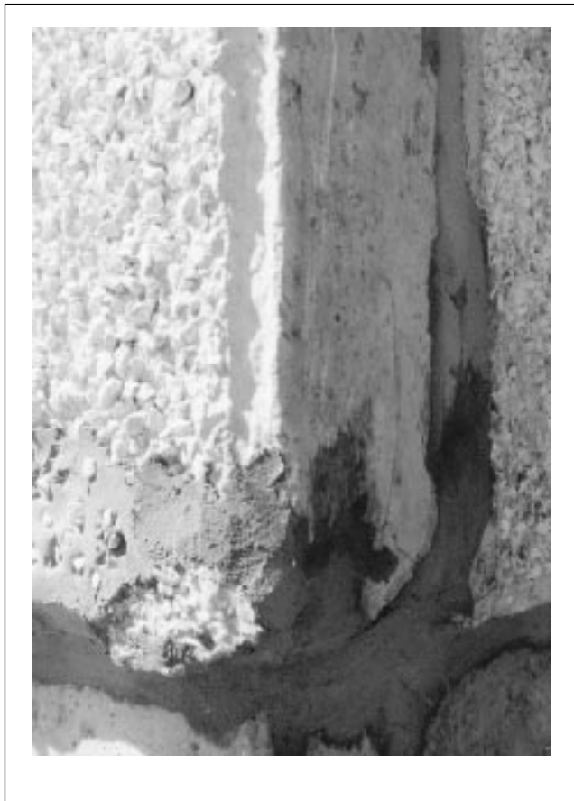
Figure 3. Detail of corner joint after grouting.
