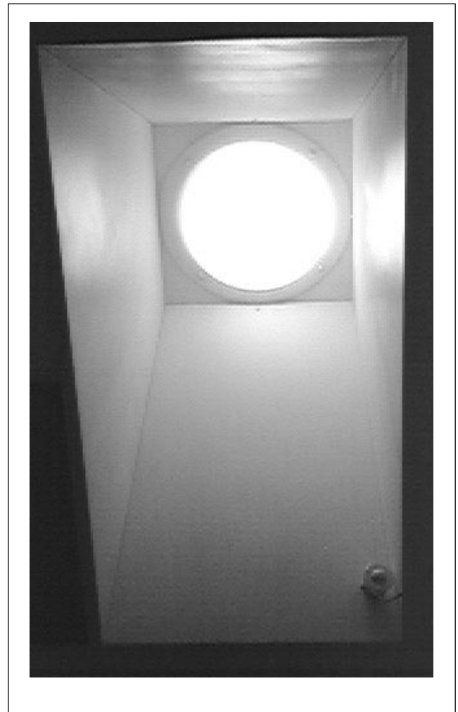
Figure 10. Auburn—Lightwell interior with repositioned photosensor
