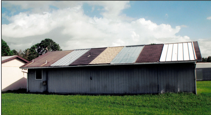
Figure 2. Flexible Roof Facility in Summer 2002 Configuration
