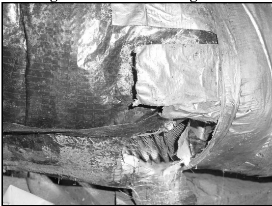
Figure 1. Before Sealing Ducts
