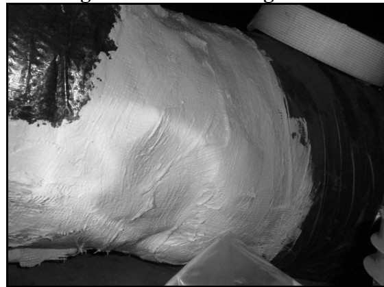
Figure 2. After Sealing Ducts
