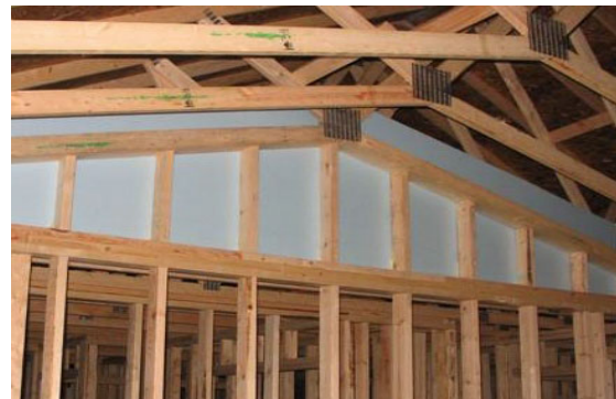
Figure 4. Attic gable wall detail
