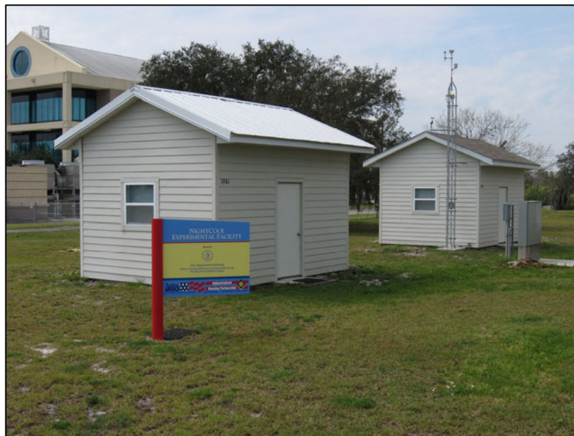
Figure 2. Completed Side-by-Side Test Buildings at Florida Solar Energy Center
