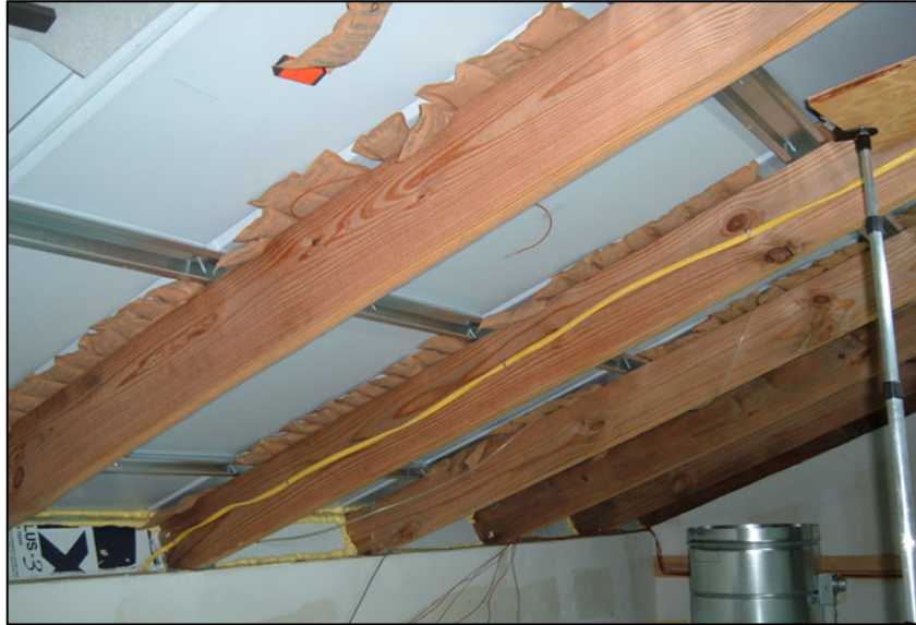
Figure 3. Interior Detail of Experimental NightCool Sealed Attic with Exposed Metal Roofing on Metal
